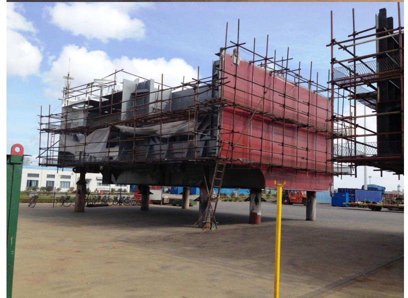
Pontoon and column block construction
