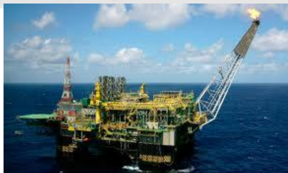
Petrobras P-52 Campos Basin
