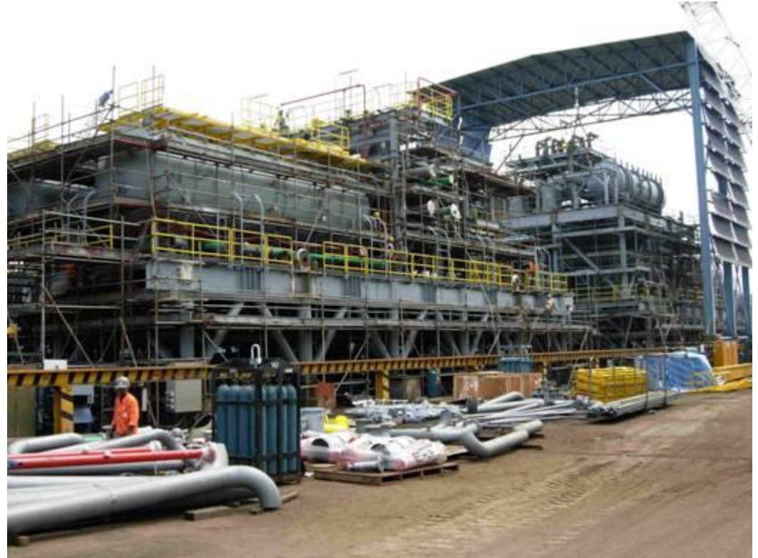
Construction of the process plant for the FPSO Polvo
